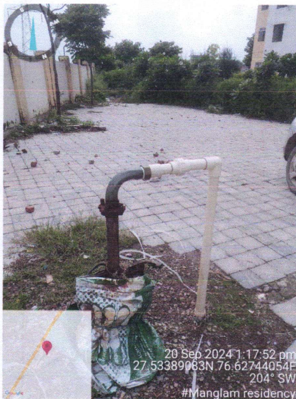
Figure 2 : Photograph of Bore Well 2 in Manglam Residency.
